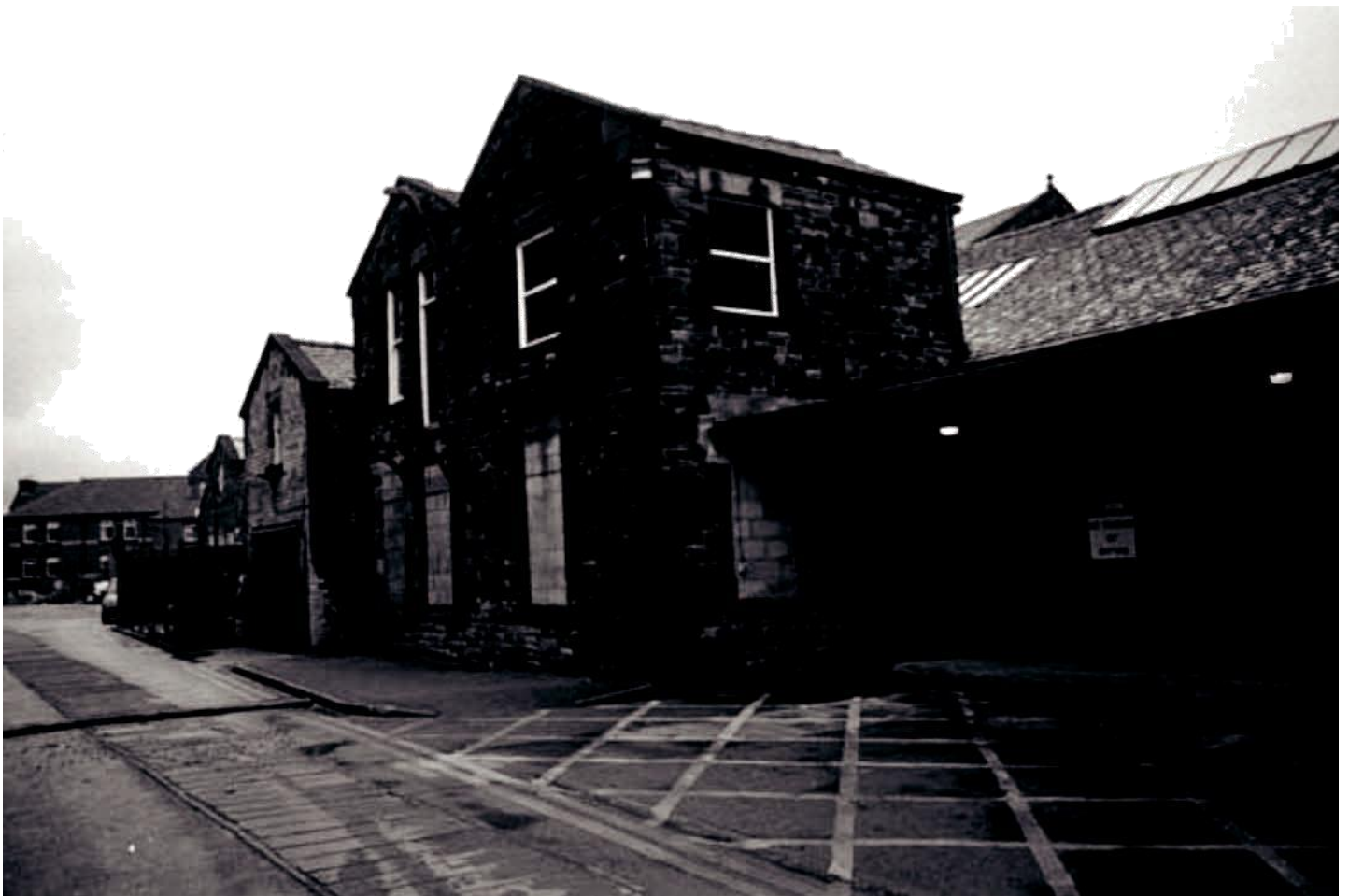
Tameside General Hospital (Ashton District). Old Ashton Union Workhouse Wing prior to demolition, October 1989. Credit: Tameside Local Studies & Archives
