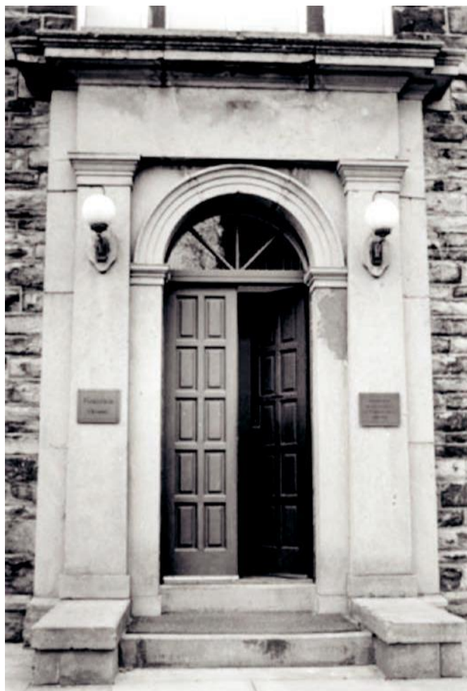
Front doorway showing brass plaque and lights, former Ashton Union workhouse, Fountain Street, Fountain House, previously part of Tameside General Hospital. Credit: Tameside Local Studies & Archives
